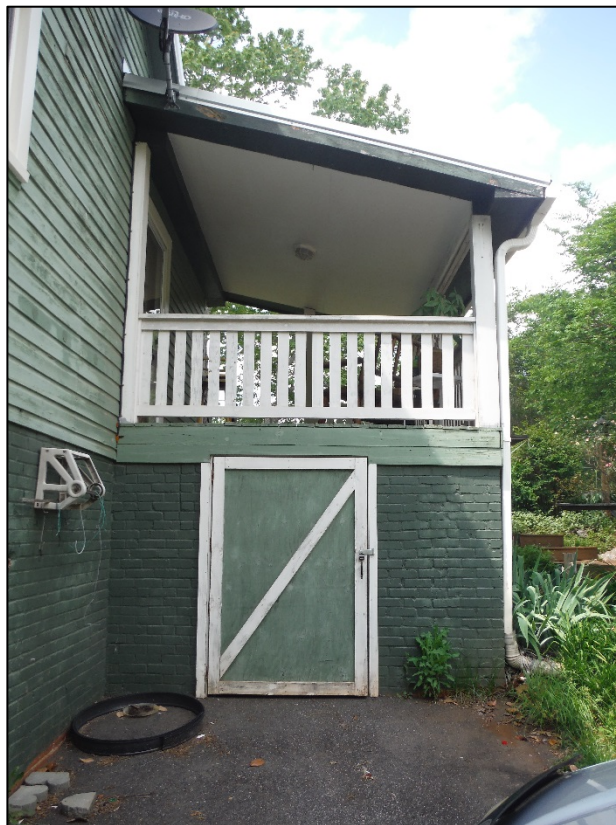
Figure 33. View of the Coggins House, below grade storage, facing north.
