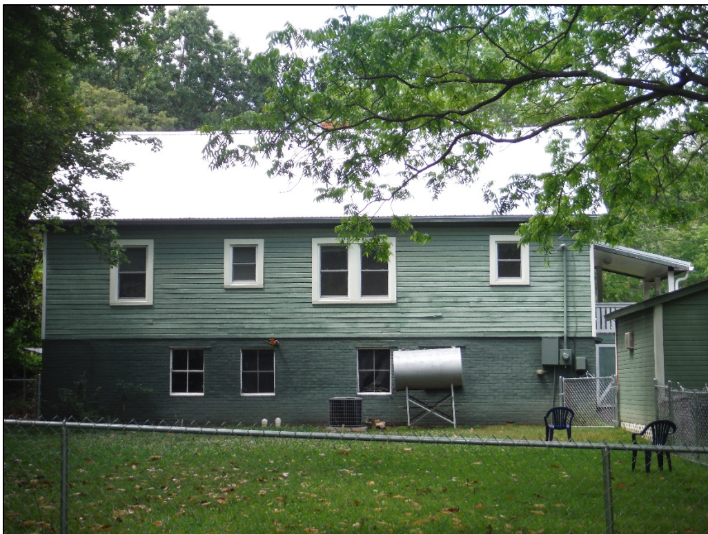
Figure 31. View of the Coggins House, facing north.
