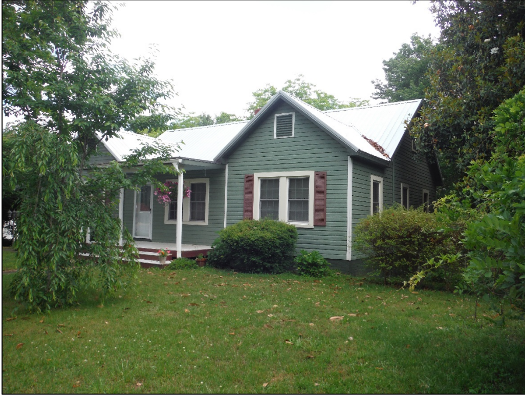
Figure 28. View of the Coggins House, facing southeast.
