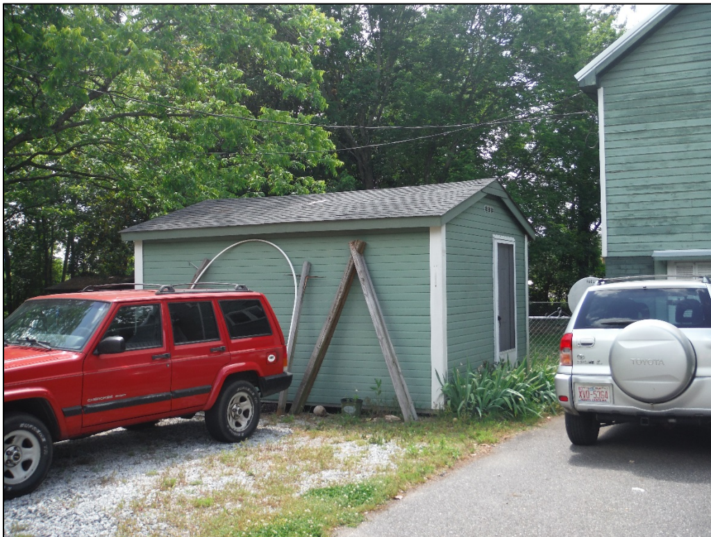
Figure 34. View of the Coggins House property, wooden shed, facing southwest.
