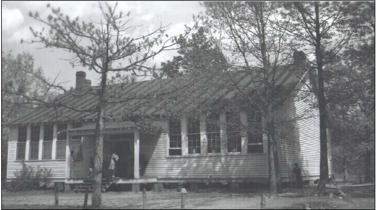
Figure 24. African-American East Flat Rock School, Henderson County, North Carolina (Fearnbach 2015:13).
