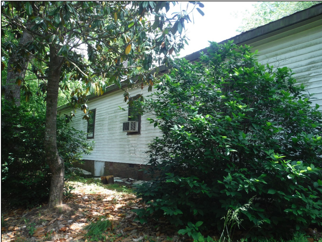
Figure 6. View of the (former) Mooresboro School, rear elevation, facing southeast.
