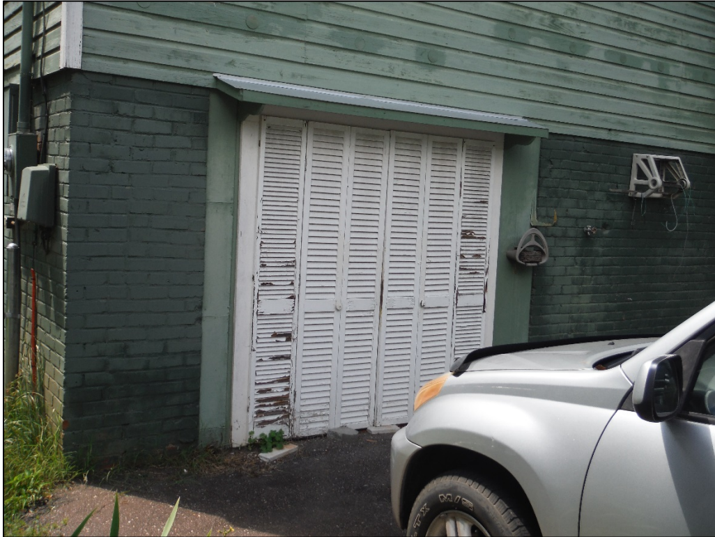
Figure 32. View of the Coggins House, below grade garage, facing west.
