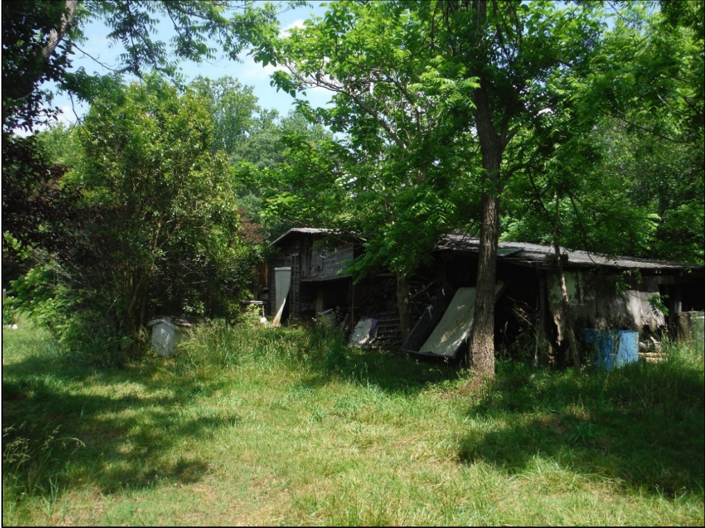
Figure 14. View of the (former) Mooresboro School property, wooden outbuilding, facing northeast.
